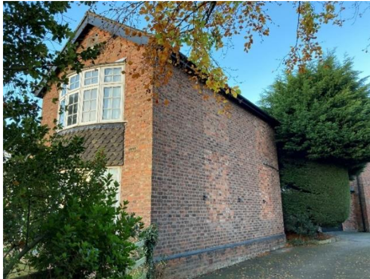
the brick chapel at Crosslooms
